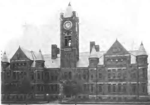
CENTRAL SCHOOL BUILDING, EAST LIVERPOOL.
